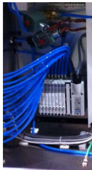
Figure 18 Pneumatic Connections
