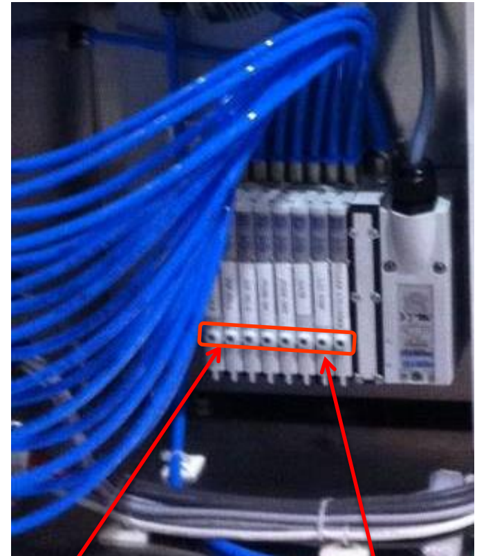
Pneumatic Air Bank Manual Over Ride Buttons
