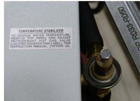
Adjustment Procedure: Loosen the lock-nut at the base of the adjusting stem of the hot gas bypass valve. Turn the stem clockwise to raise, or counter-clockwise to lower, the supply water temperature. We suggest one-quarter turn for each 2.0°F (1.1°C) adjustment. Then, wait at least 15 minutes to see if the desired temperature has been reached.
