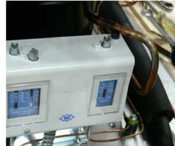
Low-Pressure Cut-Out. All platforms have a low-refrigerant pressure safety cutout. This control provides an added level of freeze-protection and serves as a low-pressure cutout of the refrigeration compressor in case of a refrigerant leak, or a restriction in the refrigeration circuit. Low-pressure cutouts will automatically reset when the refrigerant pressure increases back to normal.
